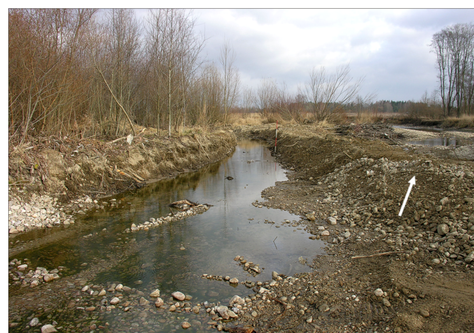
5 Re-opened inlet to a braid running inside the bend of main river channel. The arrow indicates the direction of flow along the bend of main channel. A gravelly deflector directs water to the re-activated braid and prevents it from flowing to the main channel.
